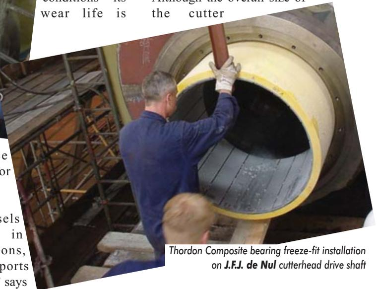
Thordon Composite bearing freeze-fit installation on *J.F.J. de Nul* cutterhead drive shaft
