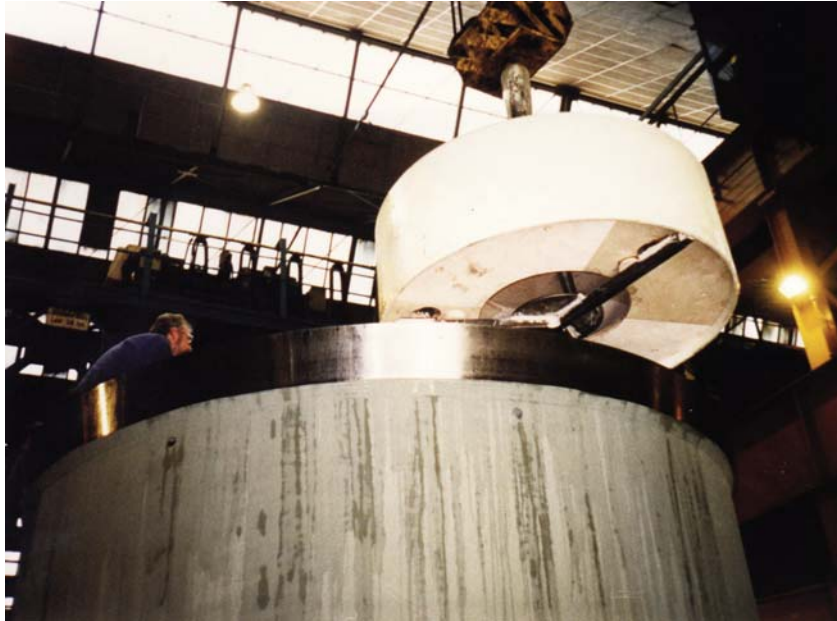
Thordon SXL bearing being installed in stern roller
