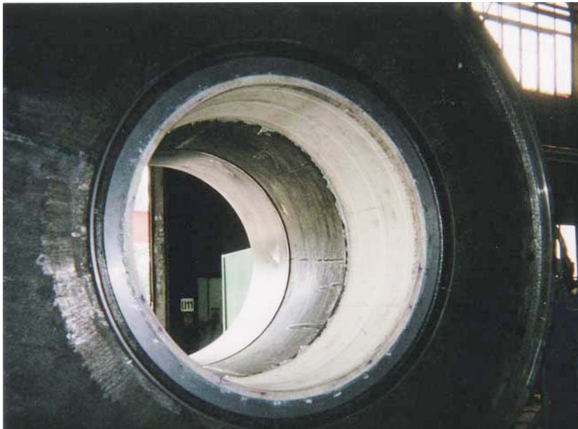
Thordon SXL bearing installed
