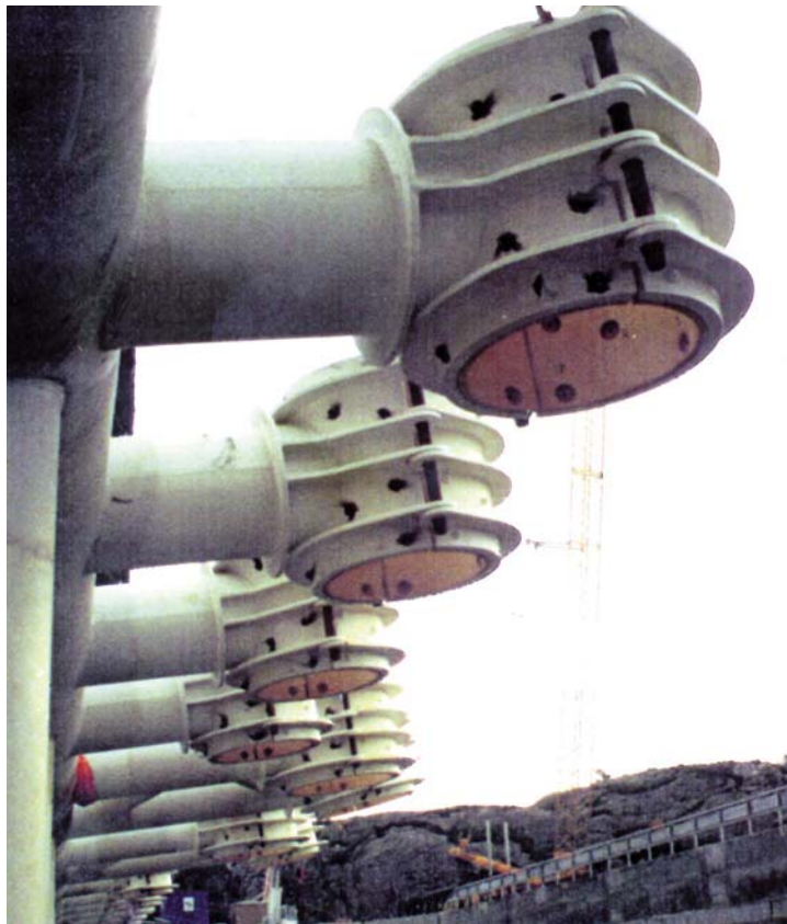
Bearing support structure
