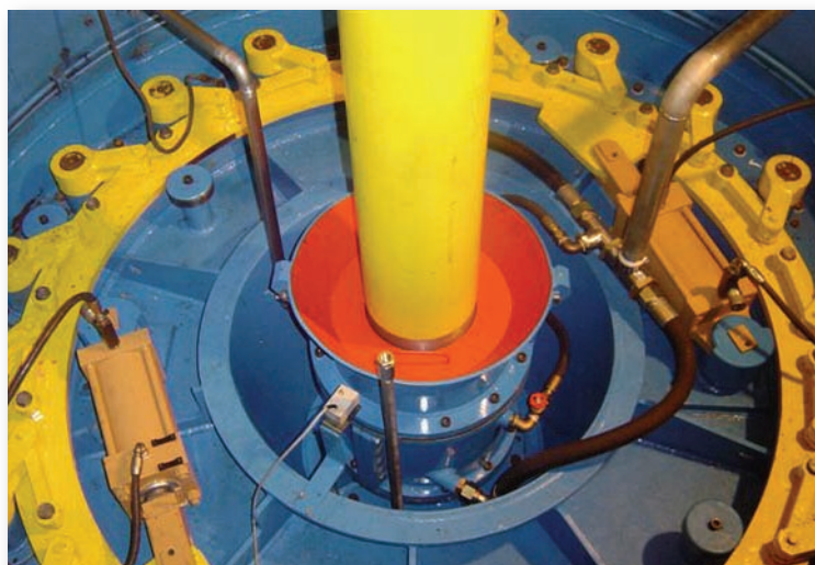
Thordon SXL main guide bearing installed at Graus Power Station, Spain
