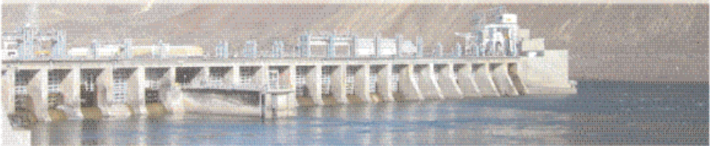
Rock Island Dam Hydroelectric Facility located on the Columbia River, Washington, USA
