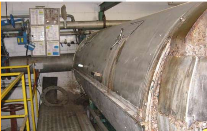
8 SXL bearings installed in trammel
